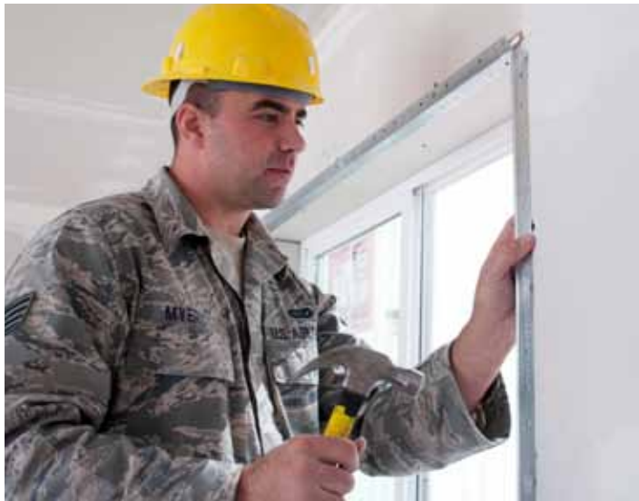
Staff Sgt. Christopher Myers, 514th Civil Engineers Squadron, hammers in a section of window framing on one of the three houses Airmen worked on while in Gallup, N.M.
